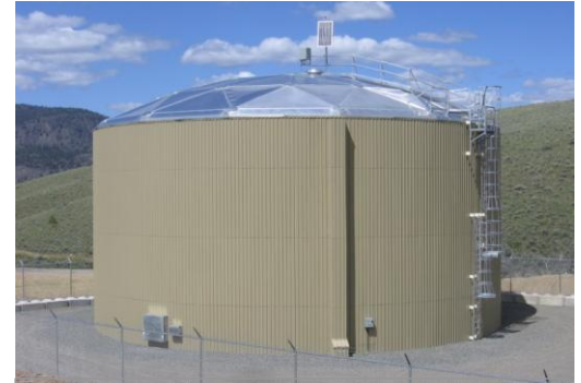
Southeast Balancing Reservoir
