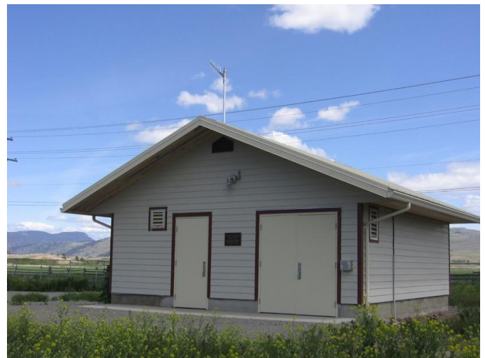
Kengard Pump House
