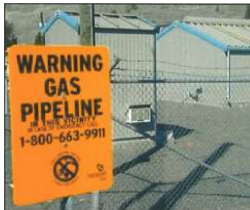
Figure 6 – Gas pipeline in the City of Merritt near the Works Yard
