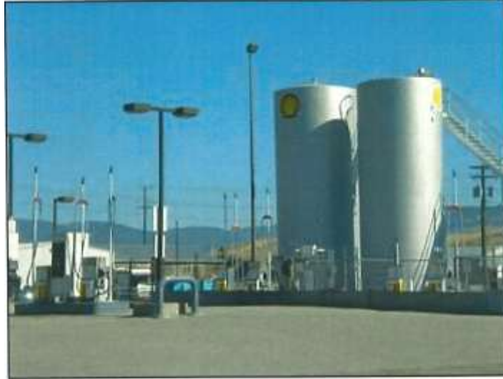
Figure 7 – Shell bulk fuel cardlock housing diesel and gasoline (Douglas St.)
