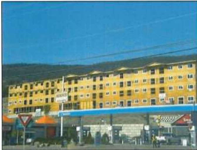
Figure 2 – Nicola Valley Seniors Residence being constructed on Belshaw St. (73 units)
