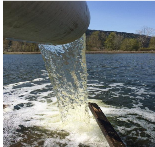
Rapid Infiltration basin
